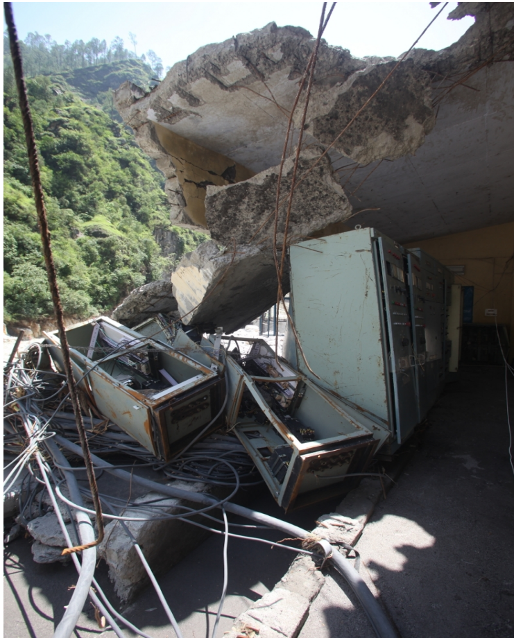
UREDA- Motigad 400KW- Electrical room- destroyed along the Paina gad.
