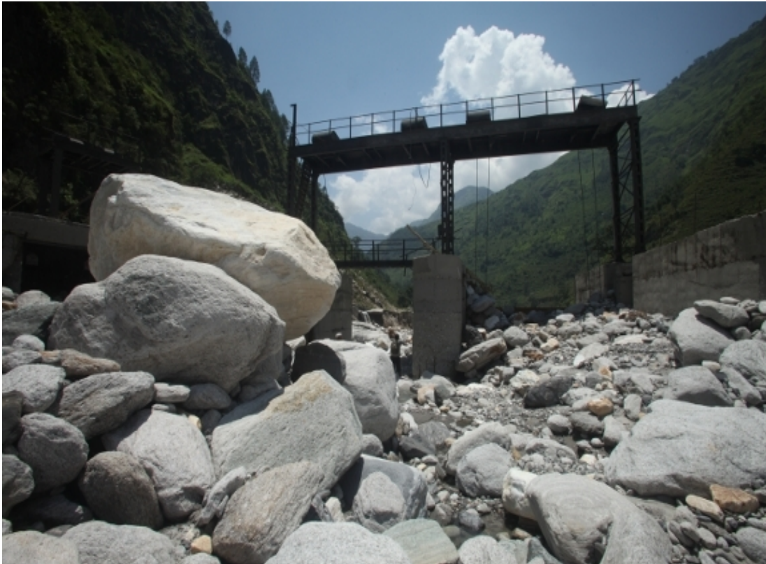
Himalaya Hydro 5 MW- Dam collapse, along the Paina Gad
