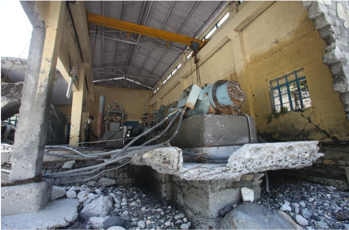
UREDA- Motigad 400KW- Power house destroyed, along the Paina gad
