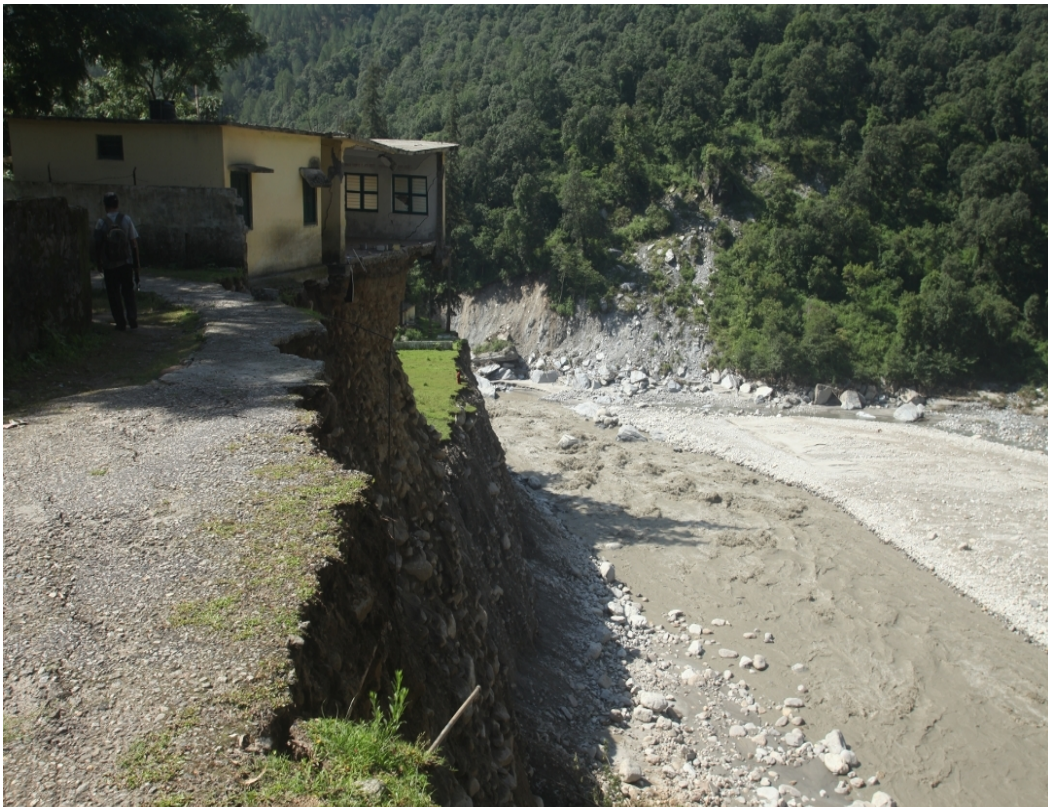
Madkot bazaar street washed away- school damaged, along the Gori river
