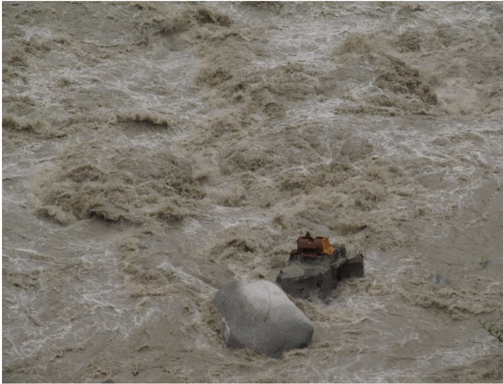
Remains of UREDA Suring gad Microhydel 800KW, in the Gori river.
