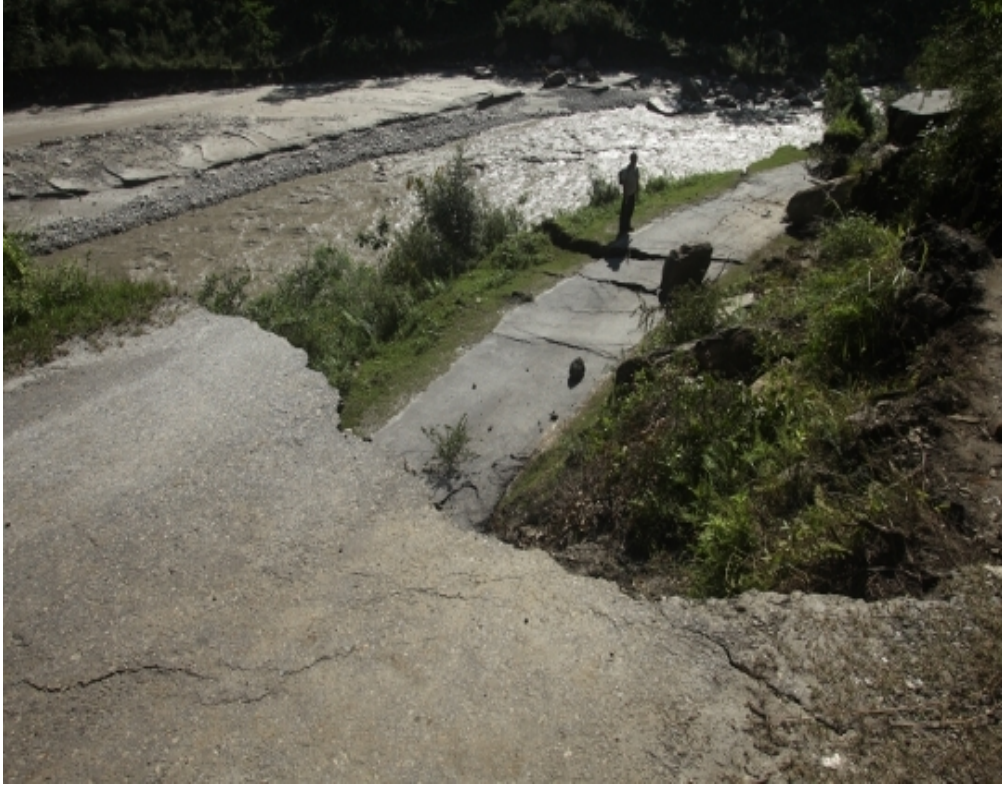
Road collapse at Bhadeli, along the Gori river.
