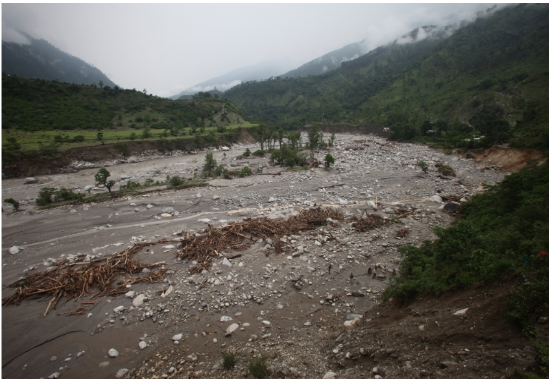
Ghattabagad road destroyed along the Gori river.
